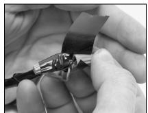
Twist the appropriate wires together, making sure that the exposed ends make good contact. Secure the wire ends with wire nuts, then wrap each wire nut securely with electrical tape to protect against moisture, as shown in the figure on the right.
